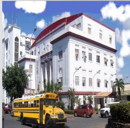
SAN PABLO CITY HALL SAN PABLO LAGUNA
