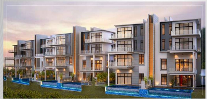
Island Resort, Batu Ferringgi, Penang Malaysia 39 units Home Elevators
