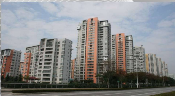
Donghulinyu Garden, Jiangsu China (20 units High Speed Elevators-32 floors, 2.5m/s)
