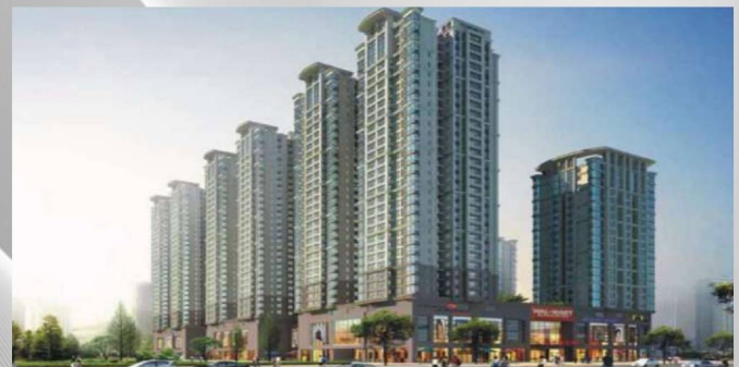
Apartment Baotou, China (17 units Elevators-32-34 floors, 2.5m/s)
