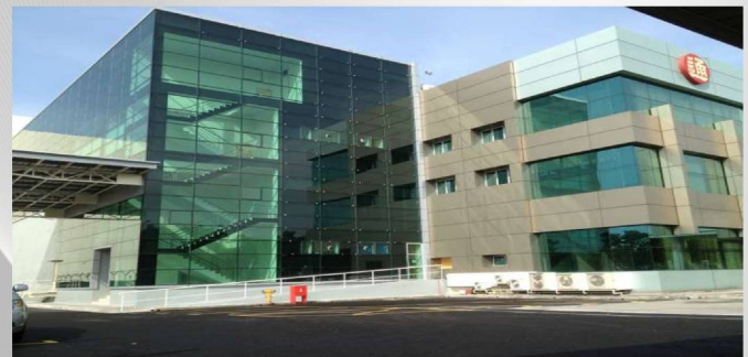
Nippon Express Factory, Penang Malaysia Forklift Elevator-4000kg capacity
