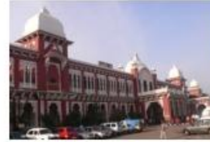
Chennai train station, India
