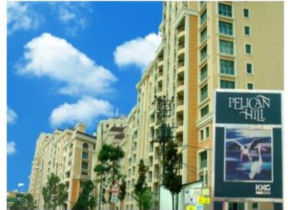
Pelican Hill Residence, Turkey.
